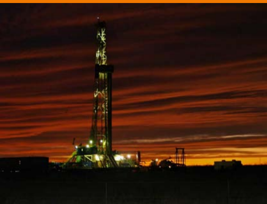
Energy development on public lands
